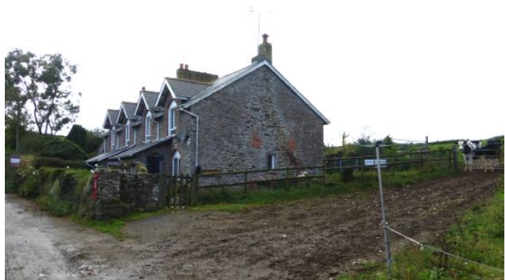
Farm workers cottages in Pepper Lane
