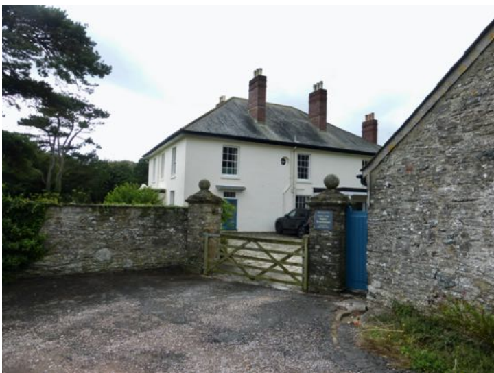
The extensive farmhouse as it stands today
